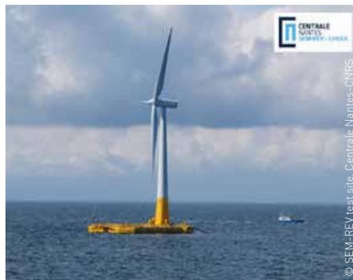
Fig. 49: Intervention at the SEM-REV test site.
