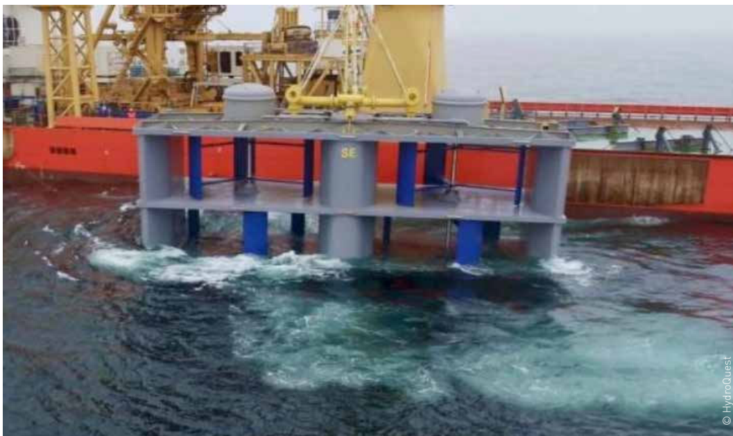
Fig. 48. Launching of the HydroQuest Ocean tidal turbine at the Paimpol-Bréhat site.
