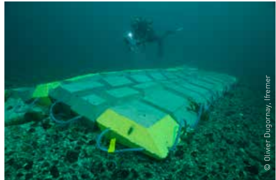
Fig. 25: Photograph of one of the monitored sites showing the cable protected by a cast iron shell and a stabilising concrete mattress.
