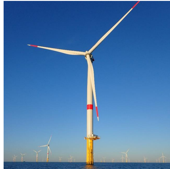
Fig. 2: Offshore wind farm off Saint-Nazaire (© France Energies Marines)
