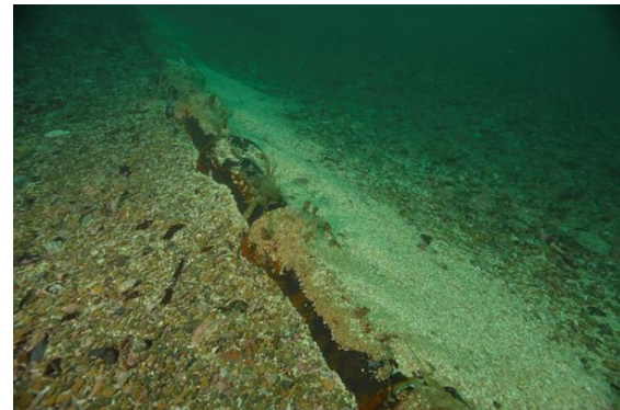
Fig. 5: Subsea cable laid on the seabed (© Olivier Dugornay, Ifremer)
