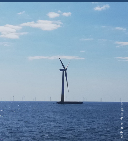
View of the Floatgen floating wind turbine in the foreground and the Saint-Nazaire offshore wind farm in the background
