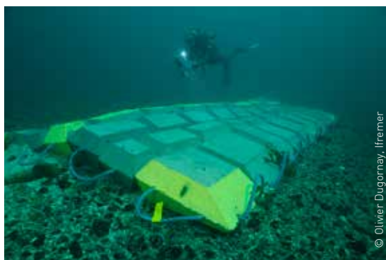
Fig. 25: Photograph of one of the monitored sites showing the cable protected by a cast iron shell and a stabilising concrete mattress.
