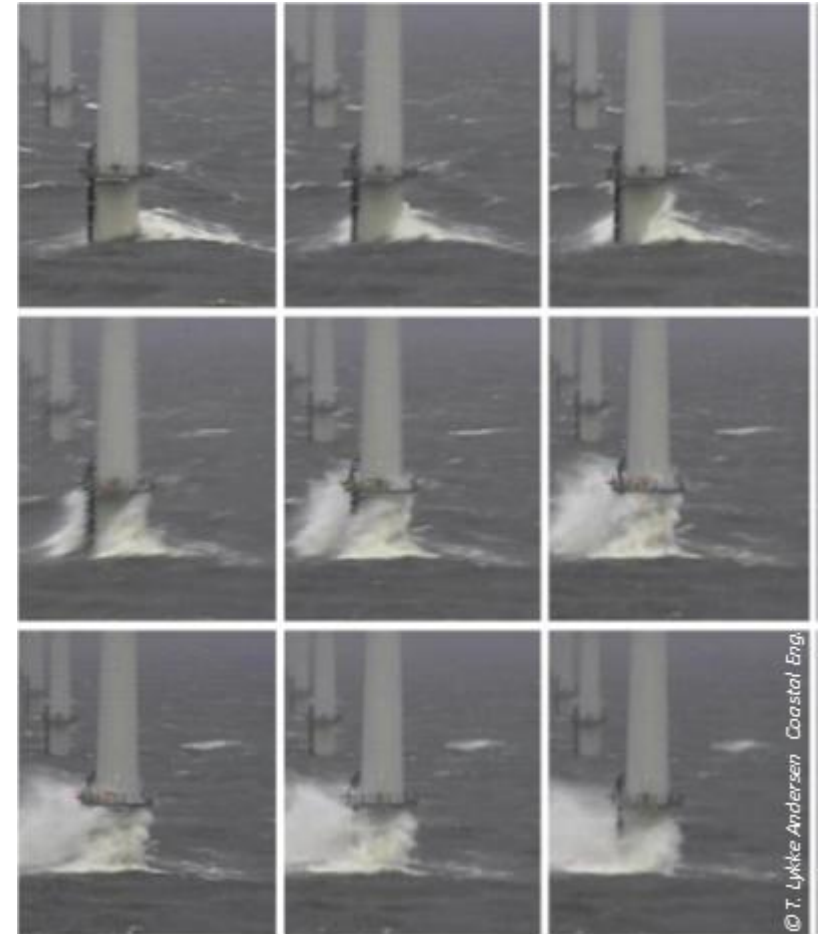
Figure: A breaking wave impacting an OWT on the Horns Reef 1 wind farm, Denmark. From Lykke Andersen et al. [2011].
