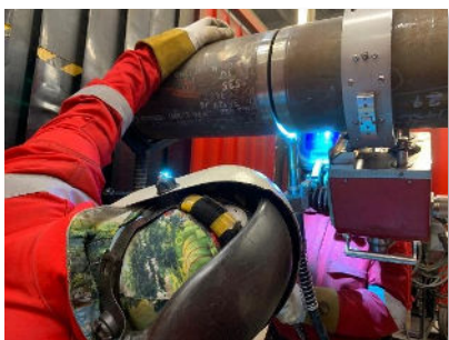
Welding for H2Pipe JIP Image courtesy of Subsea7
