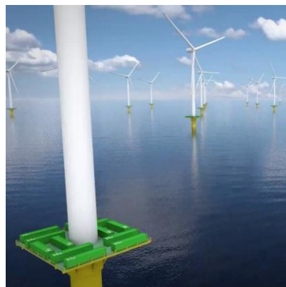
Image courtesy of Subsea7
