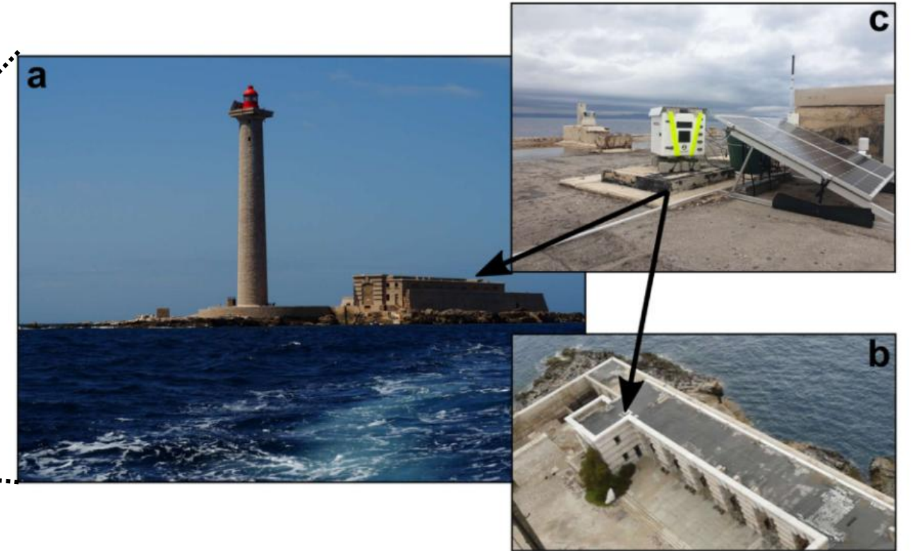
Planier island measurement station – Taken from (Thiébaud et al. 2024)
