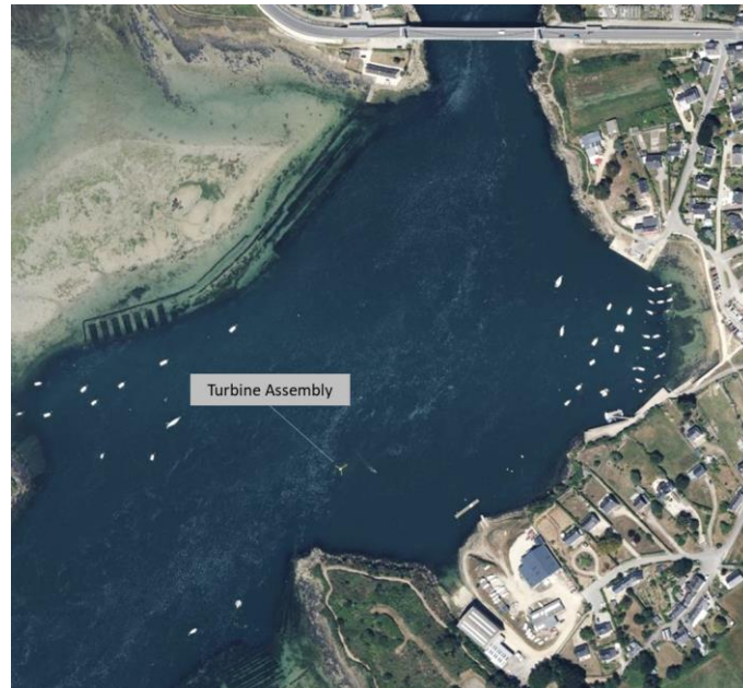
Figure 3: Turbine Position in Ria d'Étel
