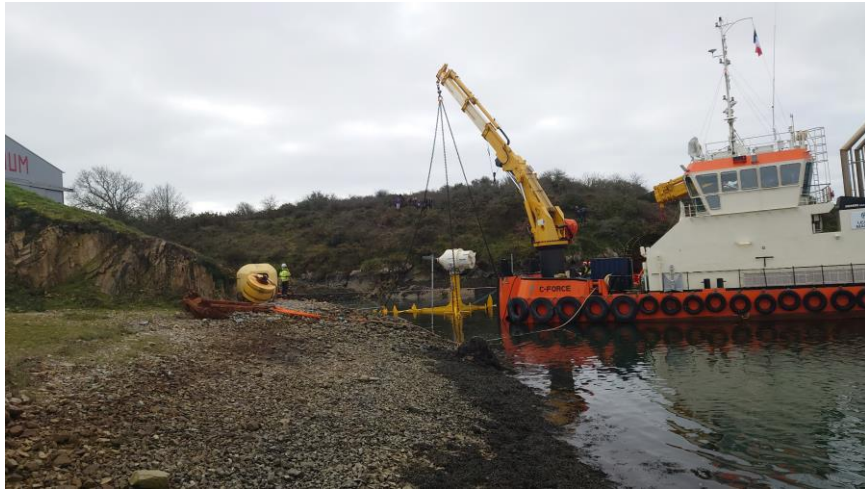
Figure 8: Multi Cat Vessel Preparing to Lift the Turbine Assembly from Slipway
