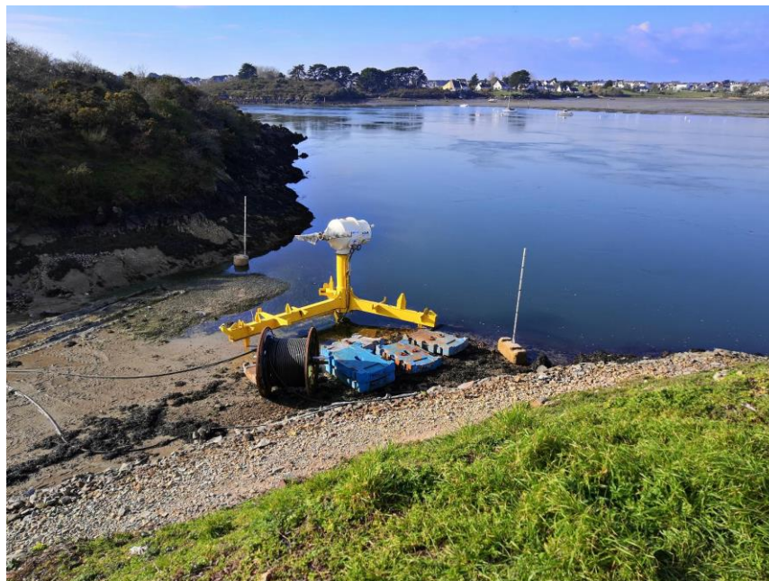
Figure 7: Turbine Assembly, Cable Reel and Ballast on Slipway Before Installation
