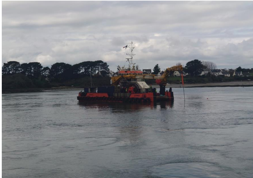
Figure 10: Vessel Landing Turbine on Riverbed
