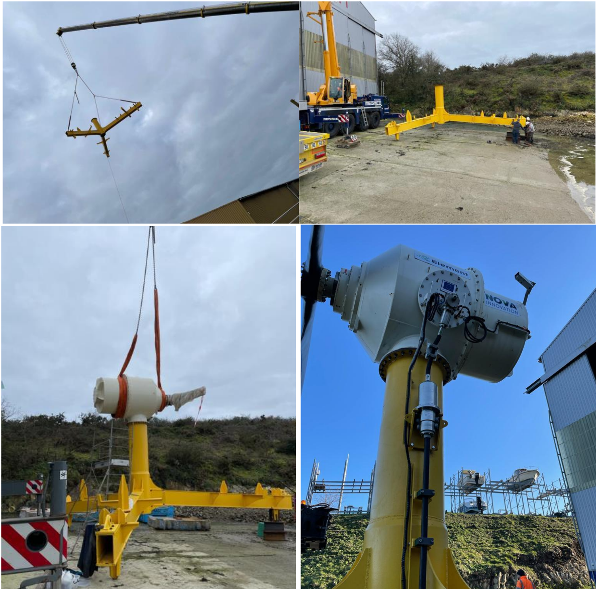
Figure 6: Substructure Lifted to CBS Slipway, Followed by Onshore Assembly of Turbine and Cable Prior to Offshore Deployment
