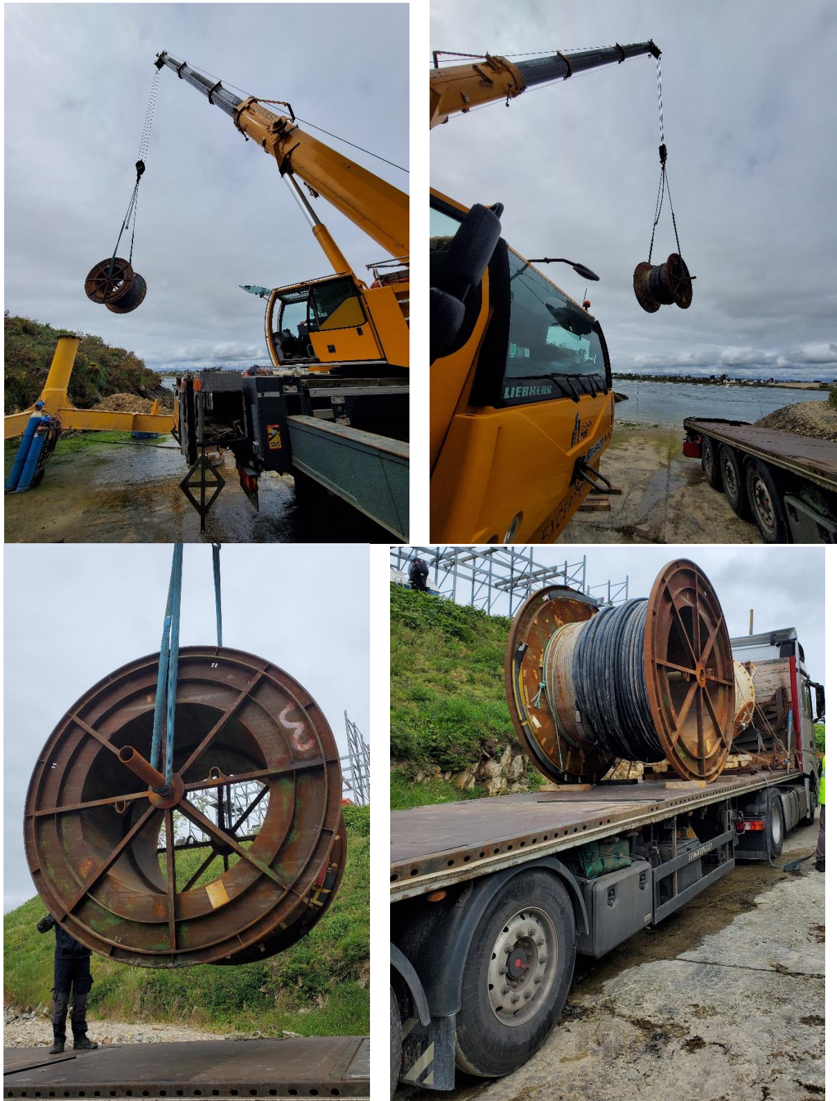
Figure 8: Moving the cable reel with the crane to the trailer
