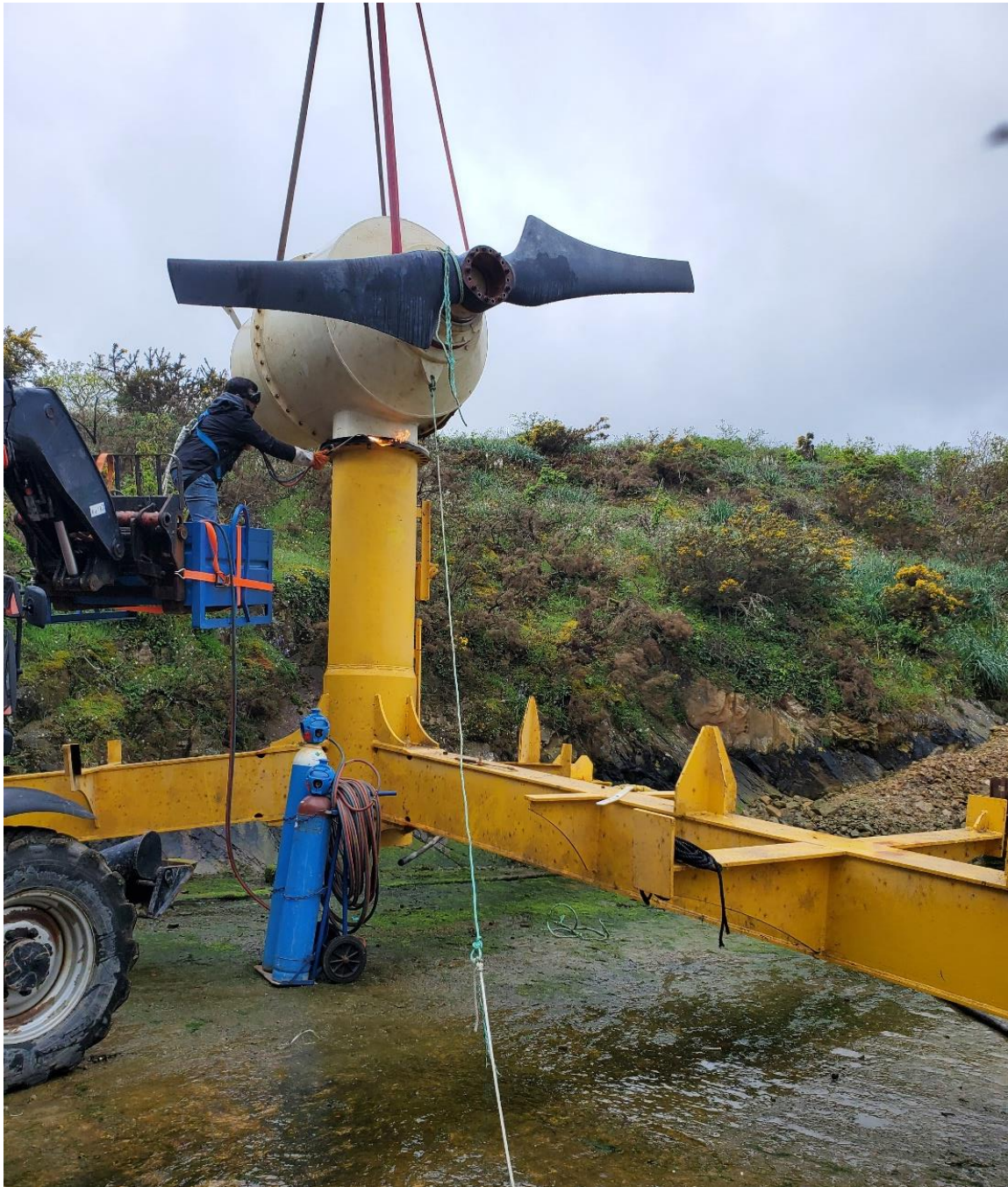
Figure 5: Heat treatment during removing the turbine from the substructure
