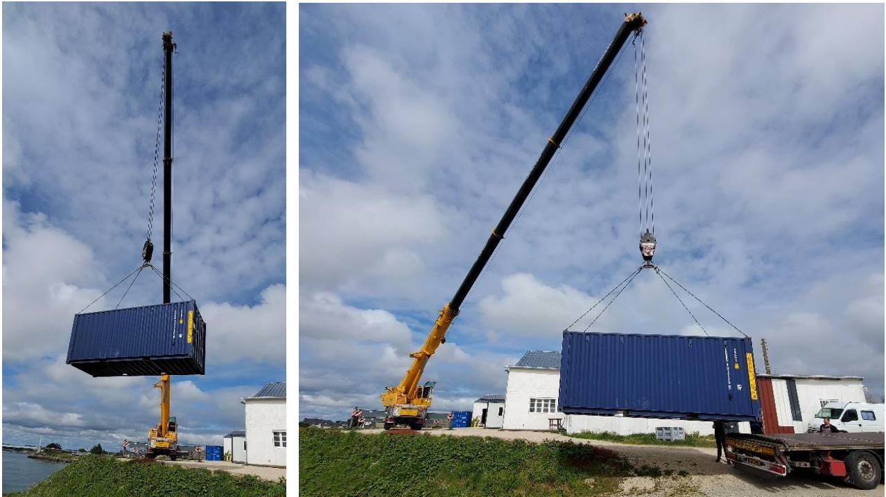
Figure 10: Moving the container with the crane to the trailer
