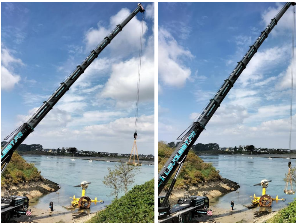
Figure 2: Moving the ballast with the crane from the slipway to the trailer
