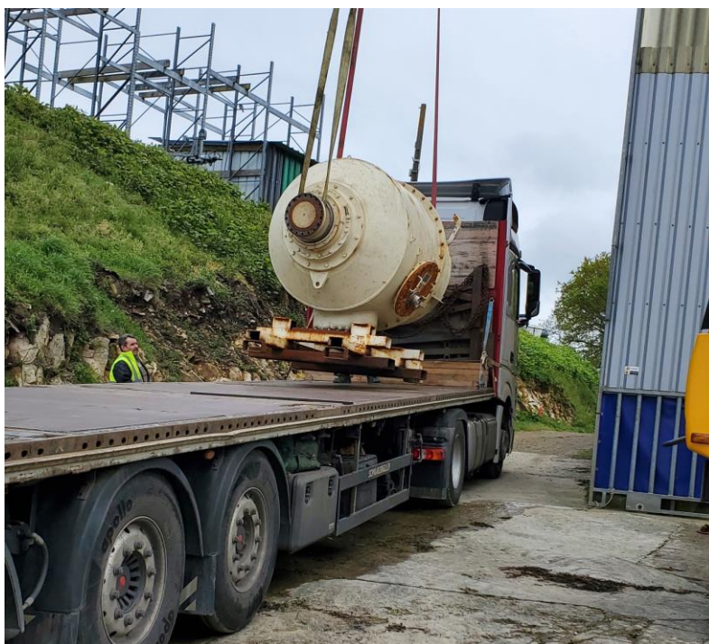
Figure 7: Moving the turbine with the crane to the trailer
