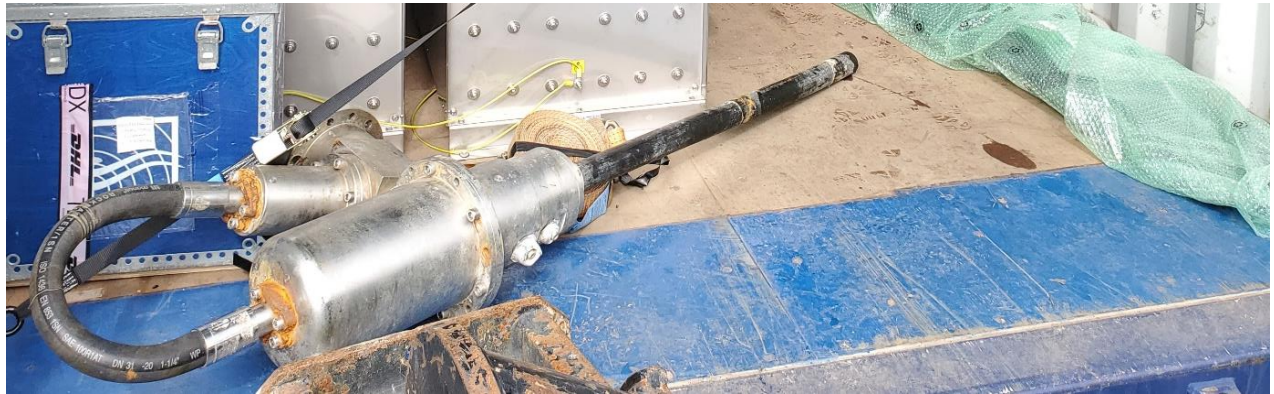
Figure 3 : The cable termination piece placed in the container
