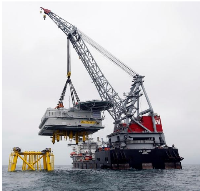
Figure 0-13: Installation of topside module onto foundation [66]
