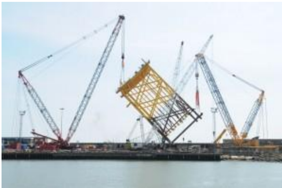
Figure 2.2.2-1: Roll-up of jacket framing [4]
