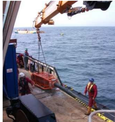
(b) dry dock connection (Wello Wave Energy device at EMEC)
