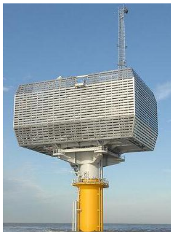
(a) monopile support structure
