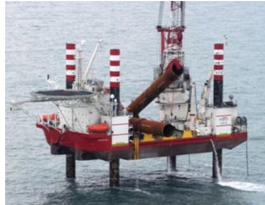
(b) lift into position [69]
