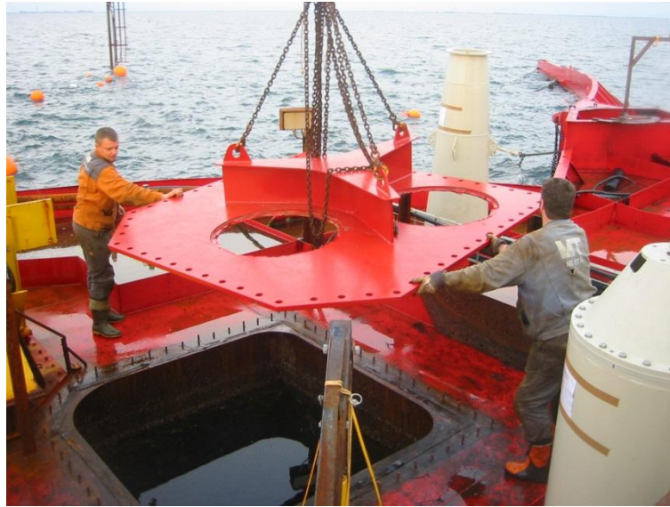
Figure 3.4.3-6: Installation of the turbine support structure (plate) [129]
