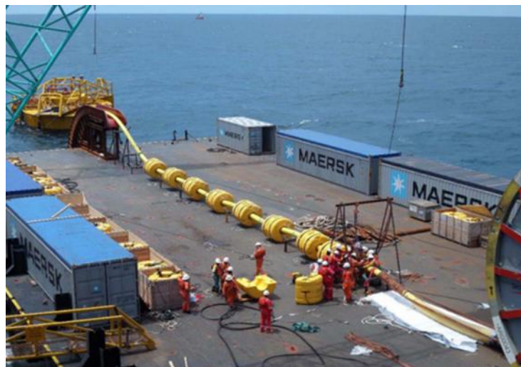
Figure 3.1.3-2: On-vessel installation of distributed buoyancy modules [46]
