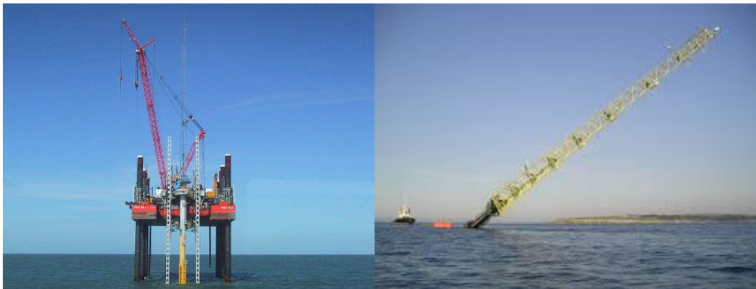
Figure 4.1.1-2: Installation of a fixed met-mast at the Rampion offshore wind farm, UK (left), towing and positioning of the IDERMAR [133] spar-buoy met mast off the coast of Santander, Spain (right)
