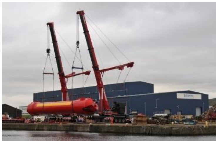
Figure 3.4.2-1: Quay wall equipped with heavy-lift crane for Pelamis tube [10]
