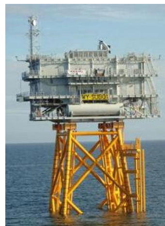
(b) jacket support structure
