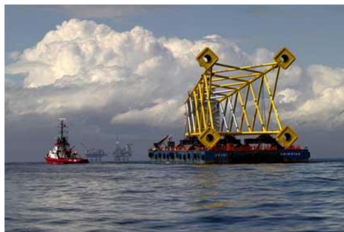
Figure 0-10: Example of post-piling Jacket structure [78]
