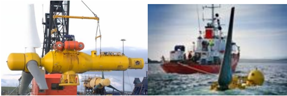
Figure 4.3.5-1: Vessel preparation for replacement of an Alstom tidal turbine [115]
