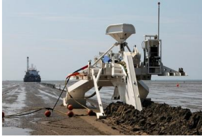
Figure 3.1.1-3: A traditional cable plough being towed [15]
