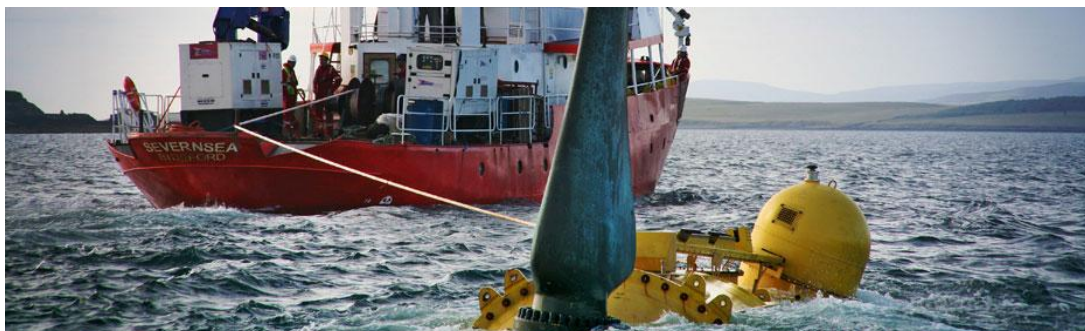
Figure 3.4.2-3: Alstom/TGL turbine towed to site [9]
