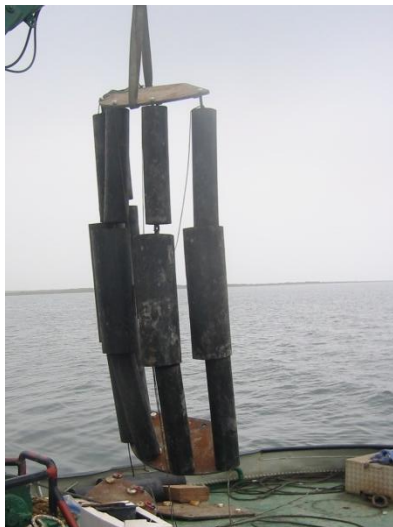
Figure 3.4.3-5: Rubber bearing lifted (left) and installed on the joint (right) [129]
