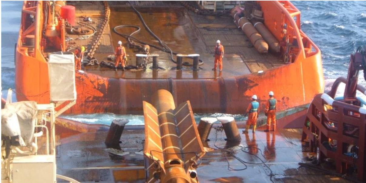
Figure 3.3.3-4: Torpedo pile being transported on deck before lowering, hanging and releasing operations into the water [87]
