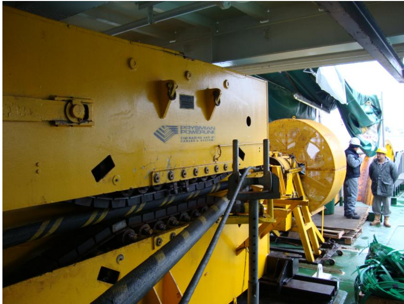
Figure 3.1.1-6 - A Linear Cable Engine used to handle offshore cable laying [15]
