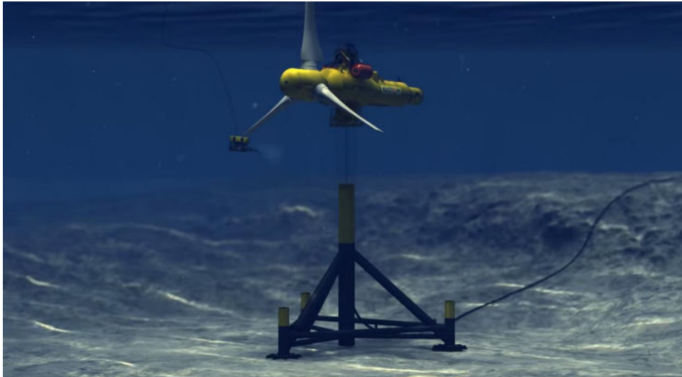
Figure 3.4.4-9: The Alstom/TGL 1 MW turbine installation procedure [9]
