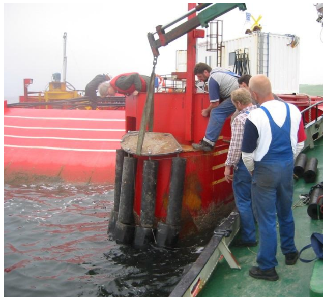
Figure 3.4.3-5: Rubber bearing lifted (left) and installed on the joint (right) [129]
