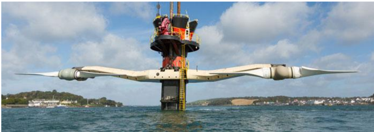
Figure 4.2.2-8: SeaGen fixed foundation tidal turbine [122]
