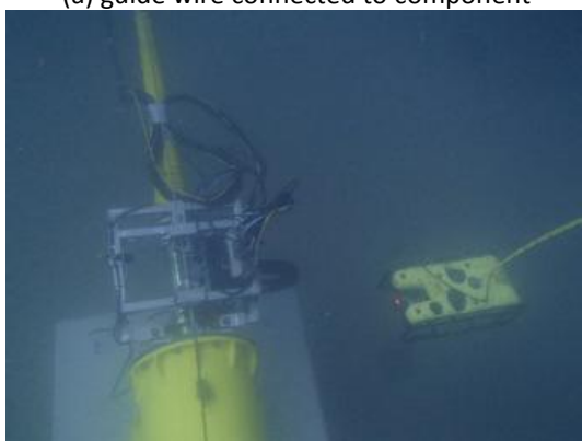
(c) cable and ROV during installation phase
