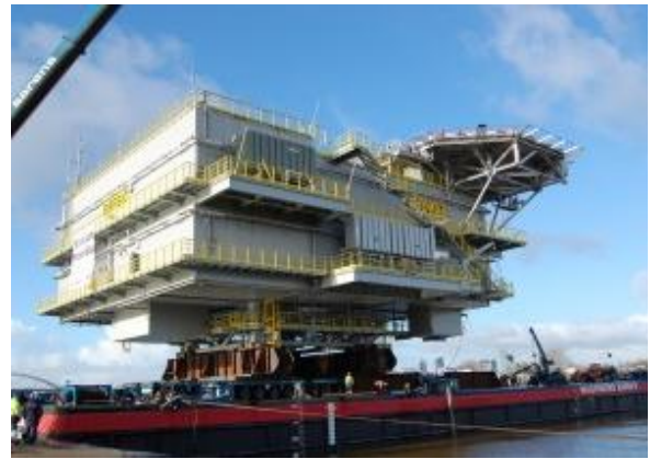
(b) topside being loaded onto barge [80].
