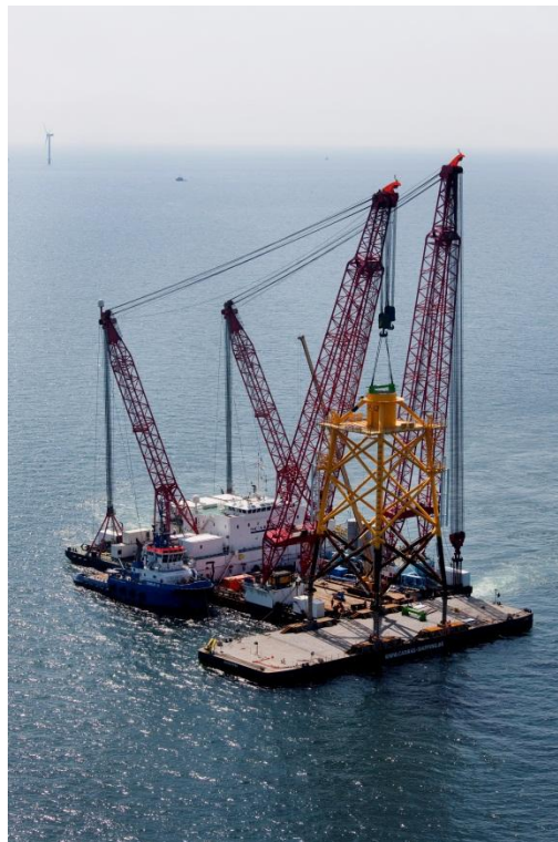
Figure 3.4.4-1: Barge with jacket foundation positioned alongside the Rambiz HLV [20]
