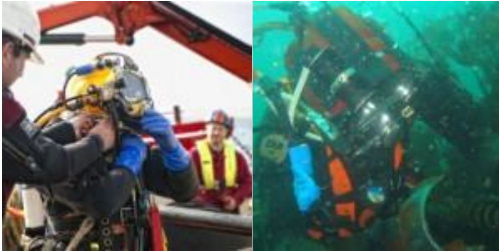
Figure 4.1.2-1: A diver preparing for subsea work (left) and diver inspecting subsea cable (right), both at EMEC [140].
