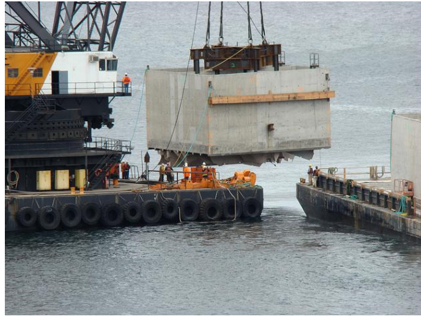
Figure 3.2.4-5: Gravity anchor being lowered into water [95]
