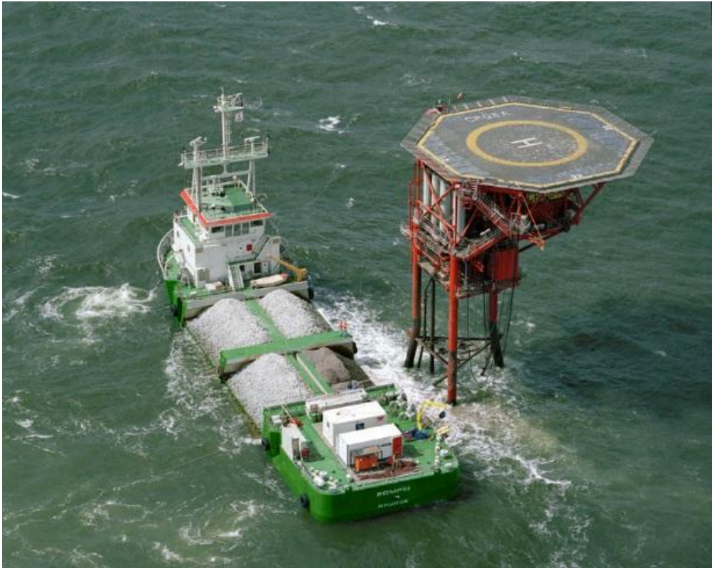
Figure 3.1.1-8: Rock placement vessel of DOME in operation [20]
