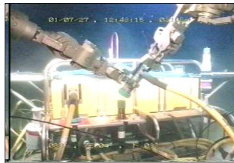
(b) subsea wet mate connection [34]
