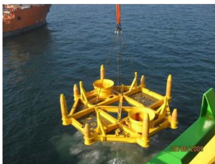
(a) pre-piling template [66]
