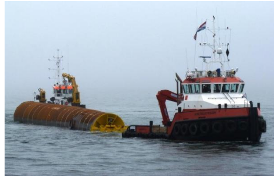
(b) capped monopile being towed [71]
