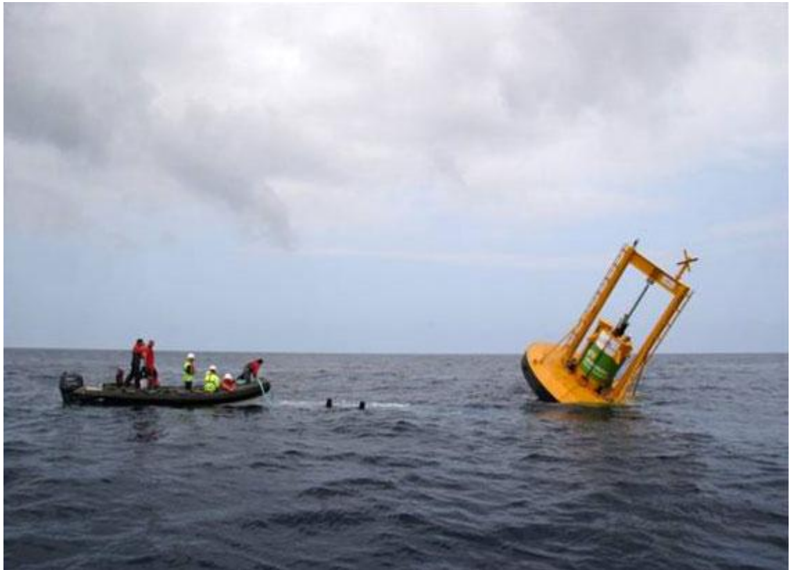
Figure 3.4.4-7: The OPT power buoy being flipped in its vertical position off the North coast of Spain through ballasting [133]
