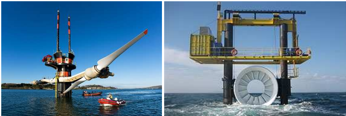
Figure 13: Piled foundation examples (left) MCT Seaflow monopile foundation system and (right) OpenHydro piled foundation system
