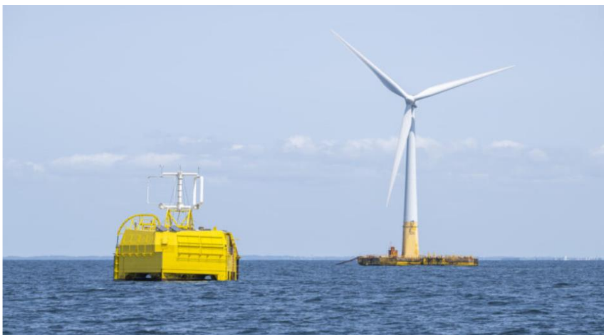
Figure 9 - The Sealhyfe offshore green hydrogen production platform.
